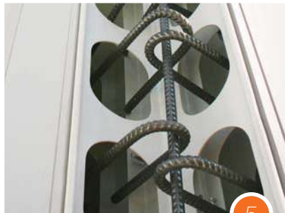
Reinforcement placement
